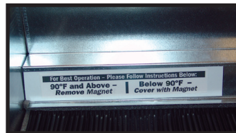
Bypass closed (normal temperature operation).
