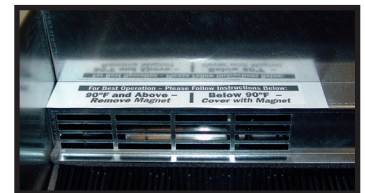
Bypass open (high temperature operation).
