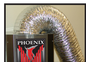
Bypass open (high temperature operation).
