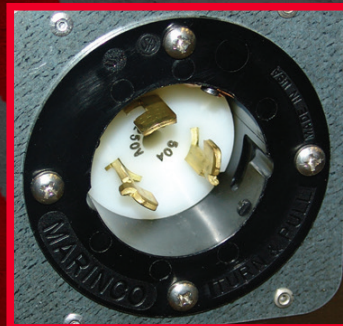
50 Amp built-in twist lock receptacle
