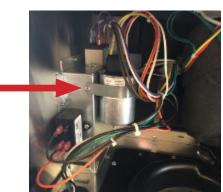
With the front cover removed, locate and remove the screw attaching the P-Clamp for the capacitor using a T20 Torx screwdriver.
