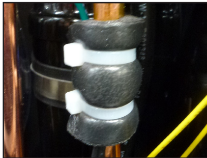
Figure 8: Thermistor attached to the refrigerant line.
